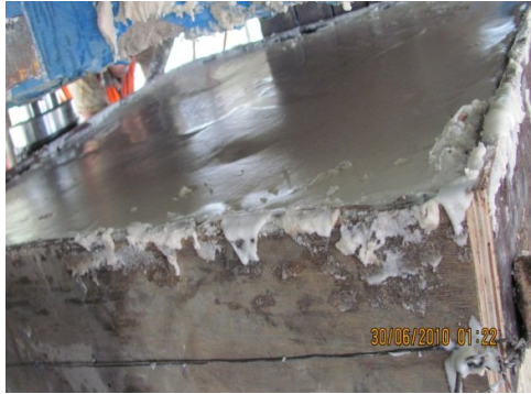
Extension of pedestal
