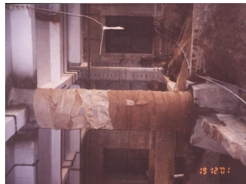
View of circular column after strengthening
