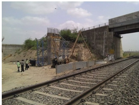
Arrangement for Dynamic Pile Test
