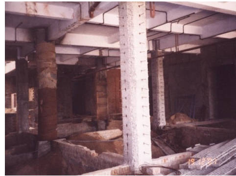
Anchor for additional reinforcement
