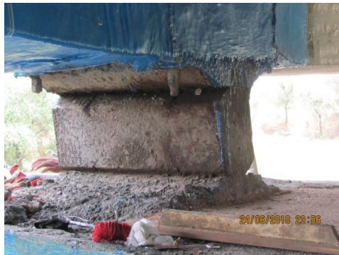
Damaged Bearing
