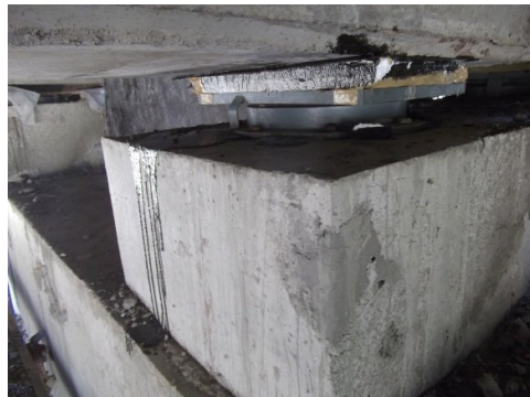
Chemical Fixing of top portion of Bearing
