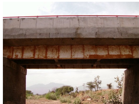
After – Strengthened Grider
