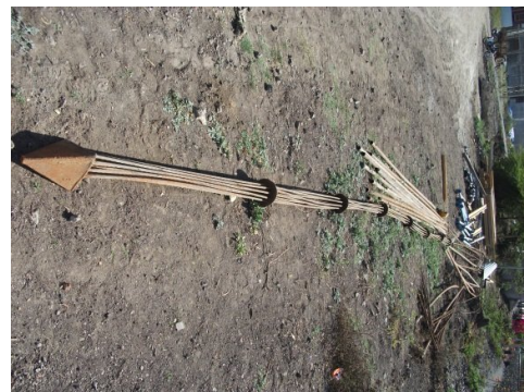
Cable for Rock Anchoring
