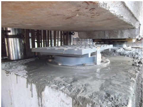
Fixing bottom portion of Bearing
