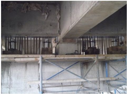
Superstructure without Bearing
