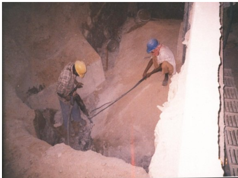
Chipping existing Foundation
