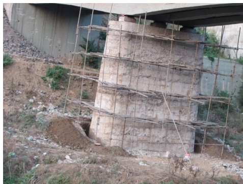
Pier having less strength – Before
