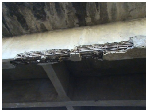
Damaged girder
