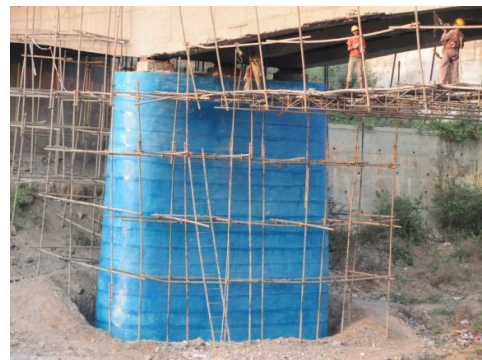
After – Strengthened Pier
