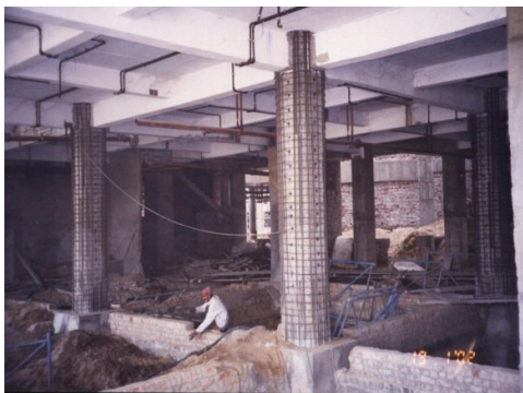
Additional Reinforcement tied to anchor
