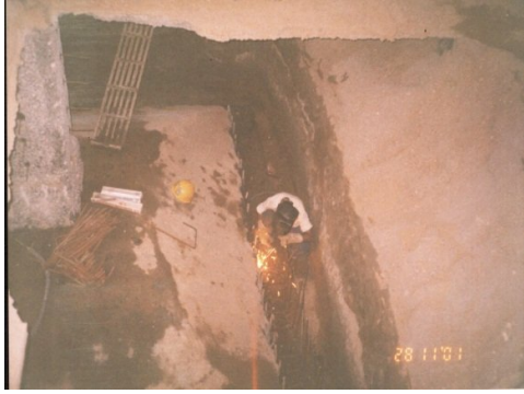
Additional reinforcement is weld with existing
