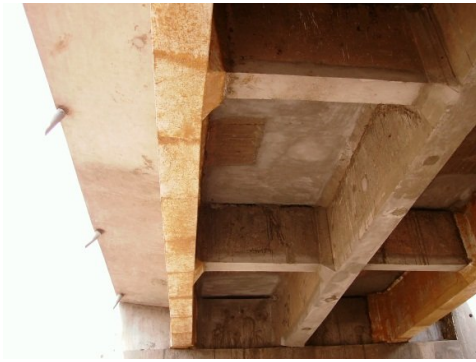
Rehabilitated Girder
