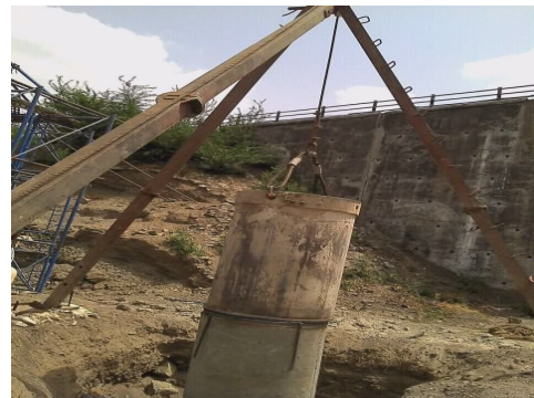
Hammer arrangement for Dynamic Pile Test
