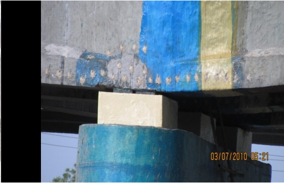
After replacement of bearing
