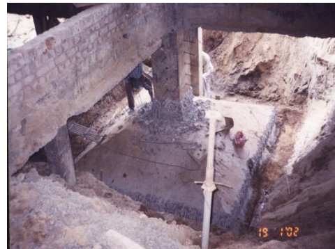
Anchor for additional reinforcement
