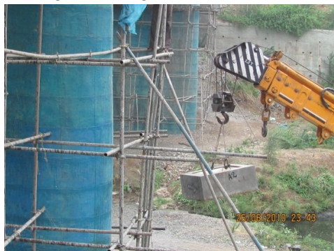
Placing of Pedestal on Pier
